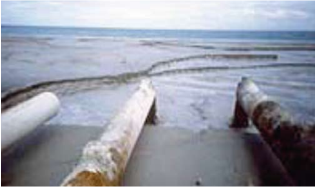
Photo 2: shows tailings pipes from the Mar copper mine in Marinduque entering the sea at Calancan Bay, Philippines
