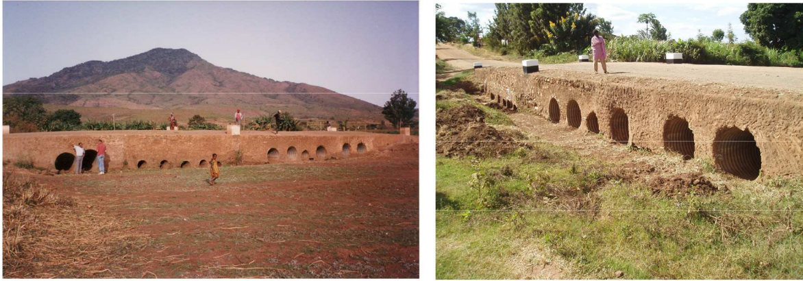
Figure 25: Flood Discharge Capacity (13 Culverts) at Kigongoni Outlet in 1991, Which Accommodated Only 25 Percent of the Estimated Flood Flow of the 1990 Flood (left). The Flood Discharge Capacity Remained Unchanged in 2005 (13 Culverts) at the Kigongoni Outlet (right).
